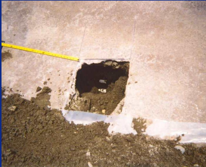
The Saw Cut – One Square Foot
